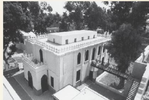
Ben Ezra Synagogue after the renovation
